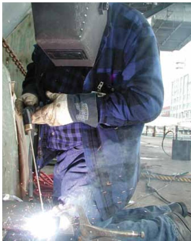
**Bremerton, WA (Jun. 8, 2002)** Wayne Weight, a shipyard worker from Paulsbo, WA, works on revamping the JP-5 fuel-overflow system on the aircraft carrier USS Carl Vinson (CVN 70). Carl Vinson is eliminating 34 of its 52 JP-5 fuel-overflow boxes and installing a more efficient pipe system. The remaining 18 overflow boxes are being replaced following an extensive deployment in support of Operation Enduring Freedom. *(U.S. Navy photo by Photographer's Mate Airman Ryan Jackson)*
